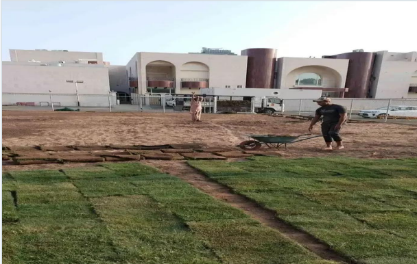
NATURAL TURF INSTALLATION
